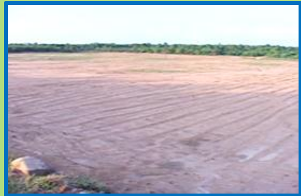
Site after back filling in oil field of ONGC Mehsana
