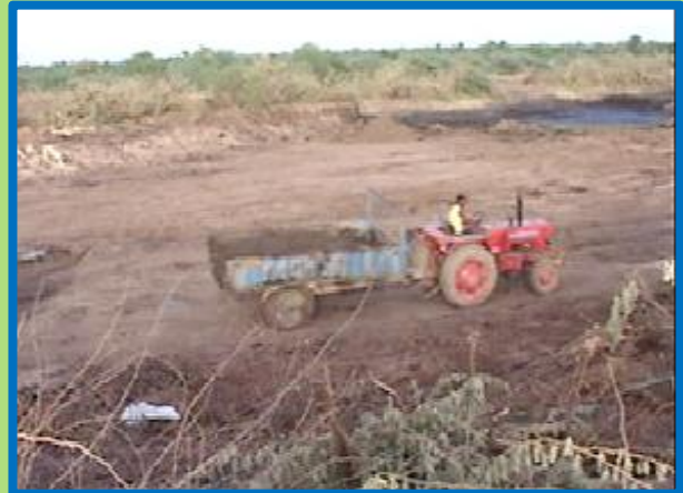
After Excavation of oil Soaked soil from Oil Spill Site
