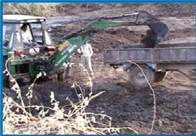
Excavation of oil soaked soil
