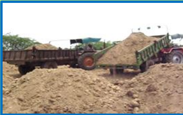
Back filling of excavated site in Oil field of ONGC Mehsana
