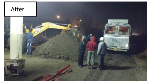
Oil Spill near WSS (Well Service Station) • Excavation of TPH (Total Petroleum Hydrocarbon) contaminated soil for Bioremediation
