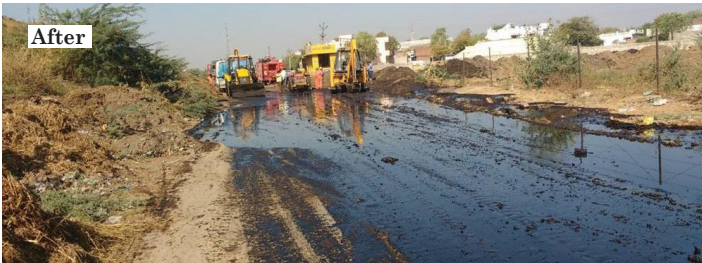
Oil Spill near WSS Recovery of liquid portion of free oil at flow line leakage point in Kalol oil field Ahmadabad Gujarat (India)
