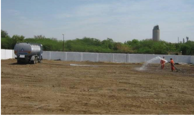
During Bioremediation Process: Application of water on TPH contaminated soil at ONGC Ahmedabad (India)
