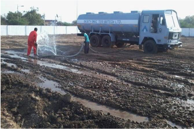
During Bioremediation Process: Application of water on TPH contaminated soil at ONGC Ahmedabad (India)
