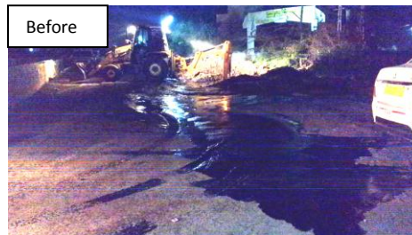
Oil Spill near WSS (Well Service Station) • Excavation of TPH (Total Petroleum Hydrocarbon) contaminated soil for Bioremediation
