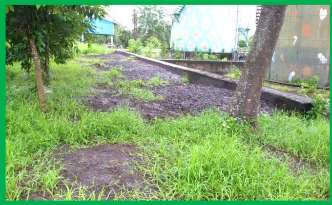
Nr. Eff. Tank 2, Before Oil-Zapper Treatment
