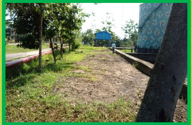
Nr. Eff. Tank 2, After Oil-Zapper Treatment
